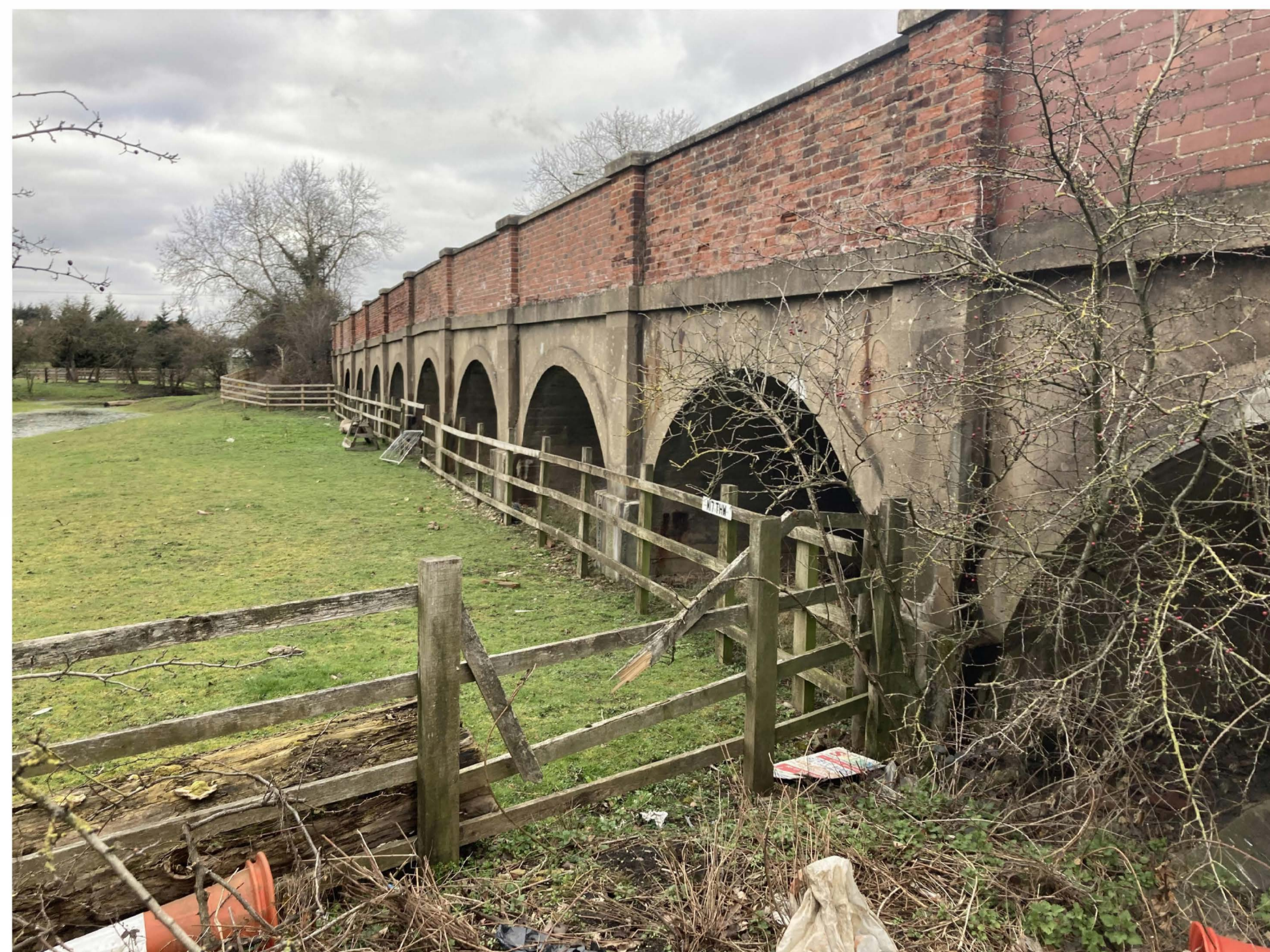
View of west side of arches
